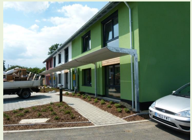
Figure 13: Flats with Brise Soleil (solar shading)
