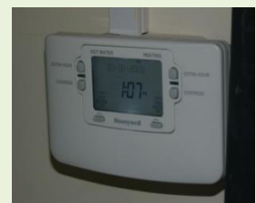
Figure 26: Boiler programmer
